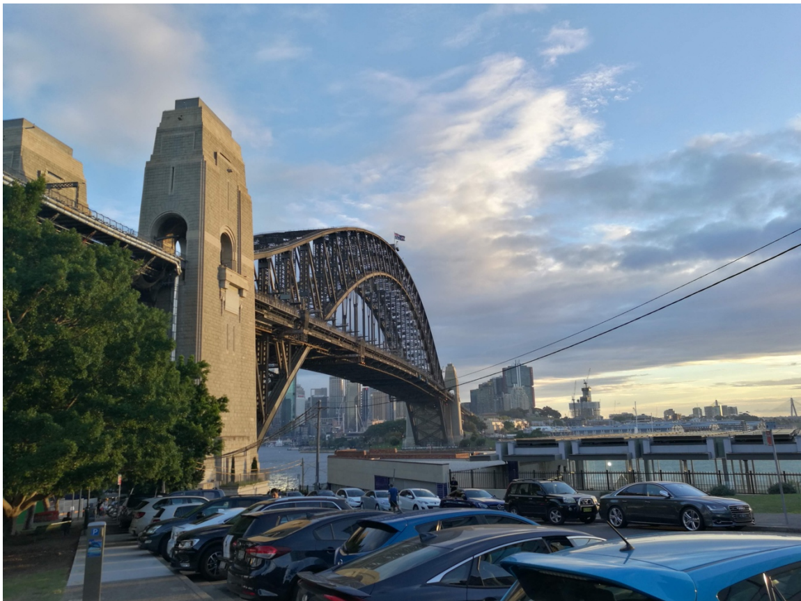
Sydney Harbour Bridge
